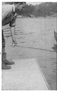
The center of lateral resistance can be verified by applying a force equal to that of the sail, by means of a line drawn in a per-
